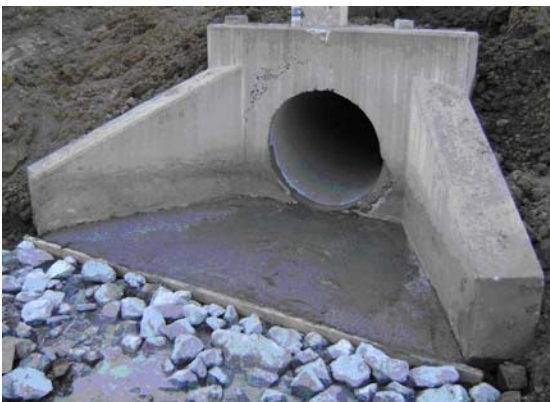
Concrete Headwall
