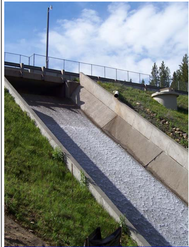
Concrete spillway on embankment of dam.
