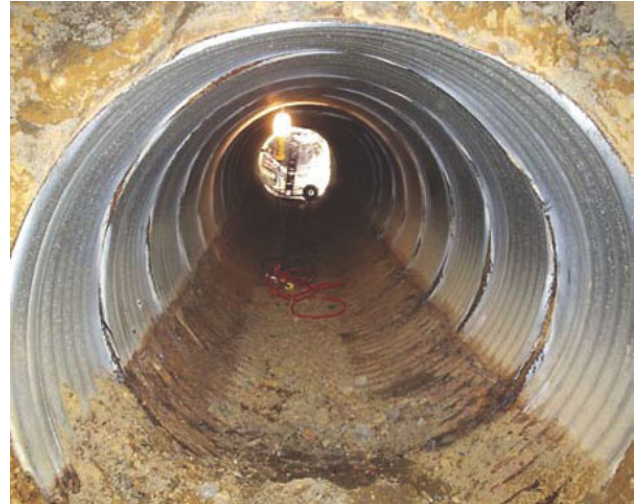
Aging metal culvert, with bulging seams and some corrosion on the bottom of the pipe.
