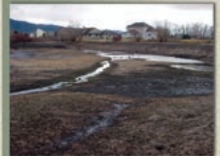
Poorly Constructed Pond
