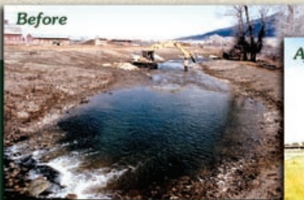
Stream restoration along the Ruby River stabilized eroding banks, reduced sediment in the streams, and improved trout spawning grounds.
